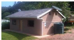
*Compressed earthen blocks do not require skilled mortar technicians to install them, delivering a faster and cheaper building process. They are bonded by the use of a liquid slurry, made from the same soil as the blocks and water. The slurry will form an unbreakable bond in 24 hours. In addition to low cost housing we have additional environmental technologies including conversion of oil sludge found in oil storage tanks.*
